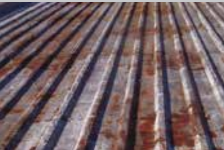
METAL RUST AND CORROSION
