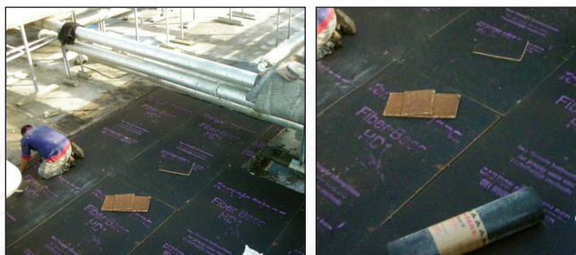
Repair substrate and any wet insulation
