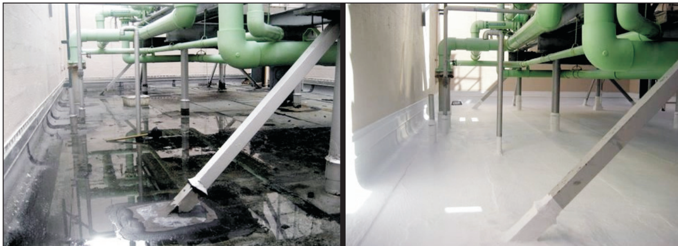
Leaky, failing asphalt substrates are converted to seamless, sustainable cool roofs.
