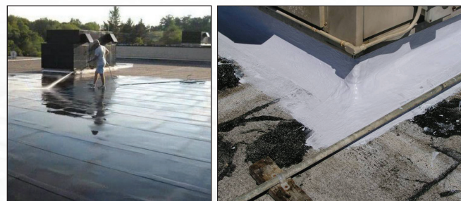
Power wash; seal curbs and penetrations
