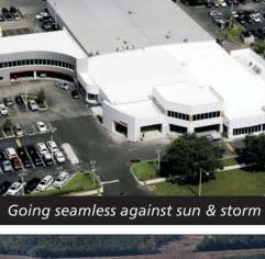
The cost was prohibitive to replace the failing metal roof of this massive 227 foot tall facility. The ASTEC® Re-Ply™ fluid-applied solution was so cost effective, five other roofs were added to this ASTEC project.
