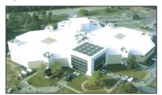
Tear-off and replacement of this EPDM museum roof was to take 4 months plus facility disruptions. ASTEC® Re-Ply<sup>™</sup> installation took 6 weeks with no disposal or interruption headaches for less than half the cost.
