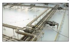
This asphalt roof with multiple supports and penetrations was a costly nightmare for traditional roof replacement, but was efficiently reroofed with a seamless, fluid-applied ASTEC® Re-Ply<sup>™</sup> System.
