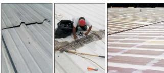
Fix wind lift & poor repairs; seal all seams
