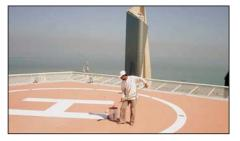
This concrete roof with a helicopter pad in Kuwait City was cracking in the hot, salt mist climate. ASTEC® Re-Ply<sup>™</sup> fluid-applied roofing bonded directly to the restored concrete, producing a single, stable and sustainable new surface.
