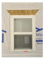
Adhere vertical sections of WindowWrap® (5A and 5B) over the jamb (side) flanges and to the shear wall or house wrap. The vertical tape should overlap the tape at the bottom and extend 3" above rough opening at the top, preferably onto the exposed sheathing.
