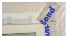
When installing arched toped windows follow steps 1B, 3 and step •4, then apply WindowWrap® Flex around arch of window.
