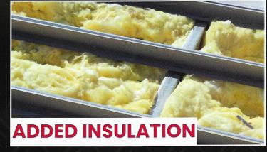
When you install Roof Huggers, the air space between the existing old roof and the bottom side of the new roof is well suited to install insulation for increasing the building's thermal resistance.
