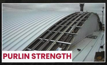
Roof Hugger Sub-Purlins Have The Ability To Add Strength To The Existing Purlins. This Is Important Because Most Retrofit Systems Just Add Weight.
