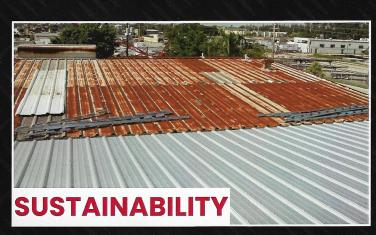
Roof Hugger's retrofit system is a sustainable solution for upgrading old metal roofs. By allowing the existing roof to remain in place, the system reduces construction waste sent to landfills.
